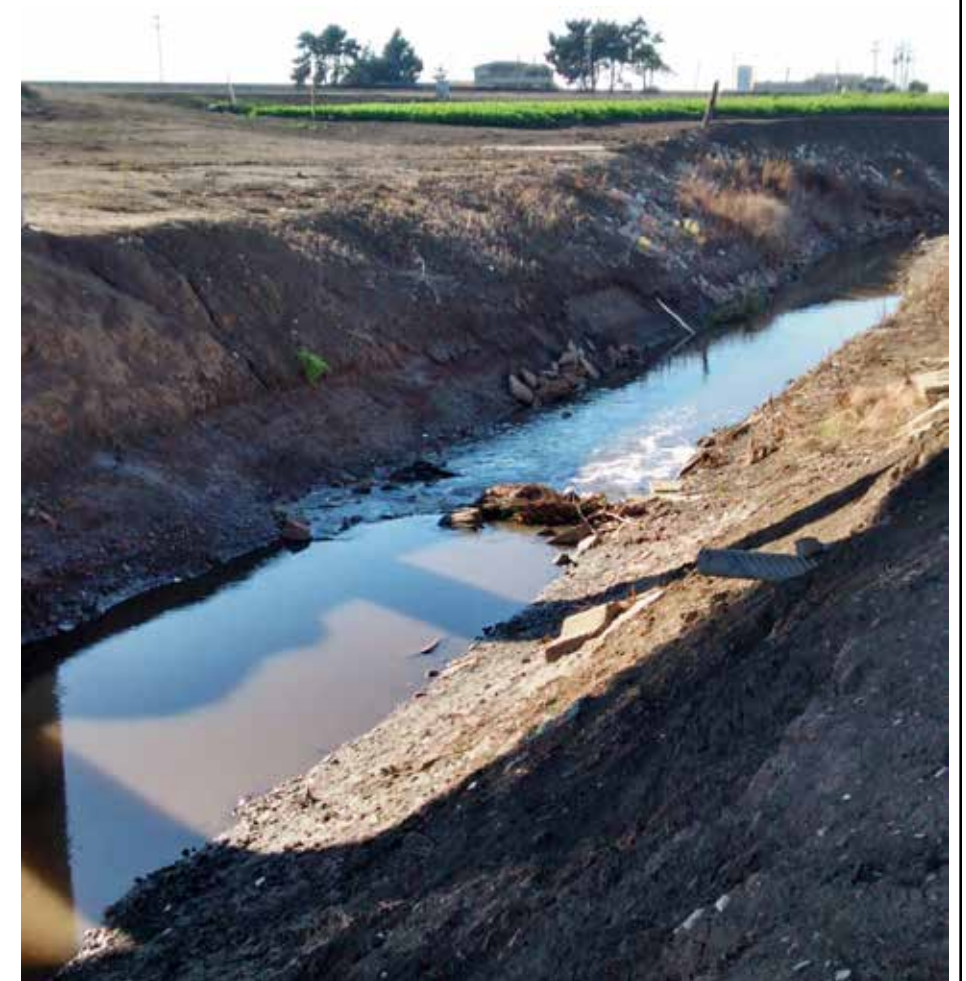
Near Reclamation Ditch Intake Site
