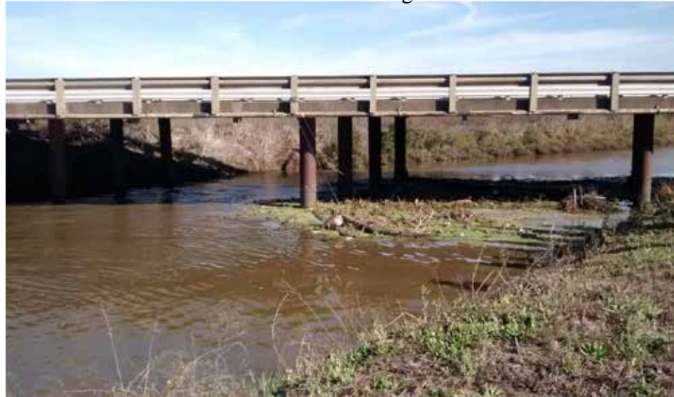
Molera Road Bridge
