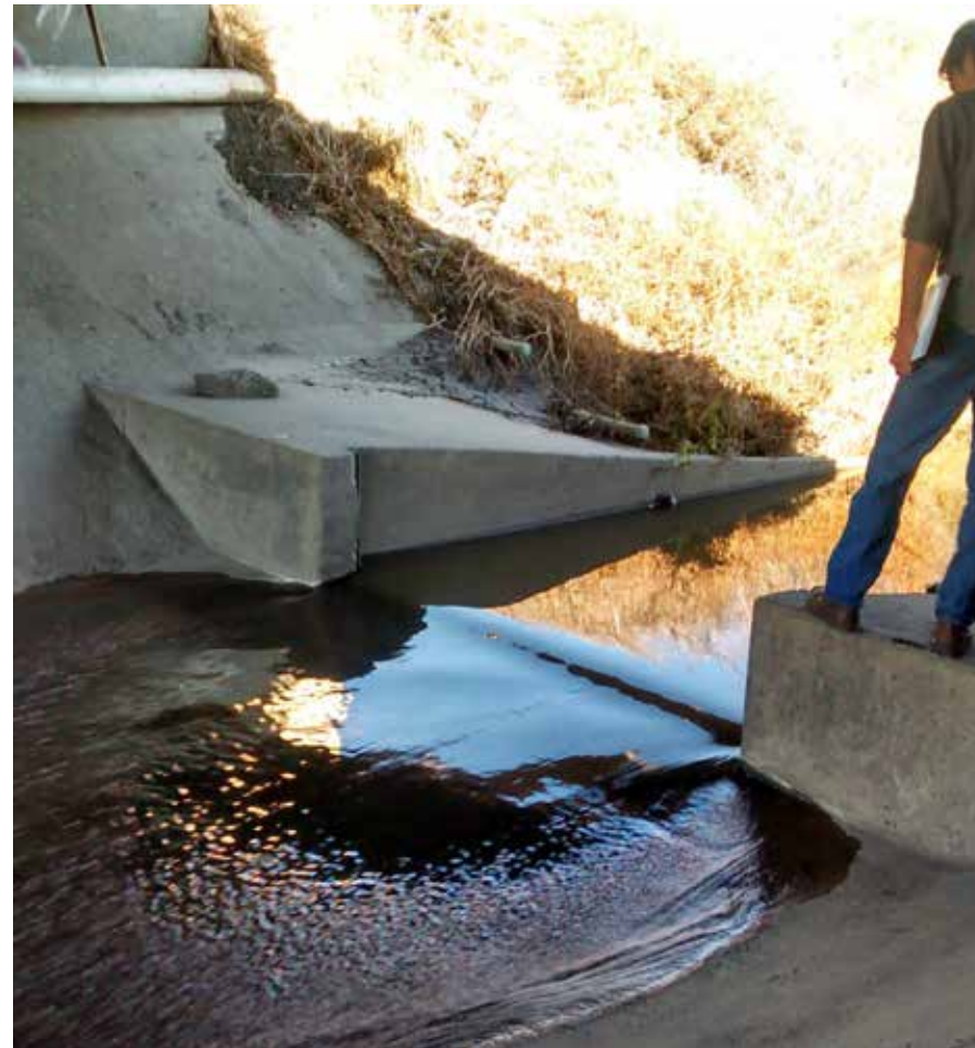
The San Jon Road Undercrossing
