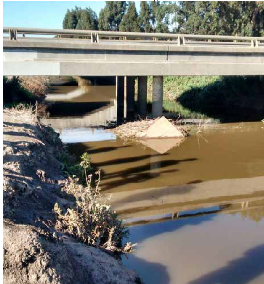
Haro Road Bridge
