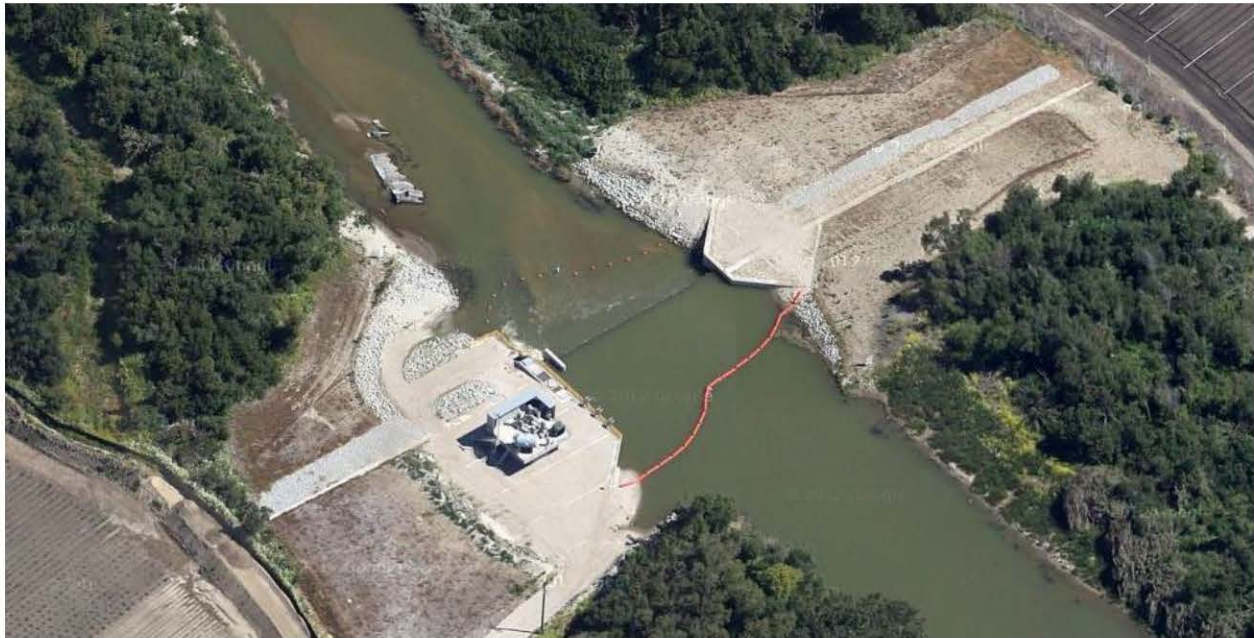
Figure 2.4: Salinas River Diversion Facility 15
