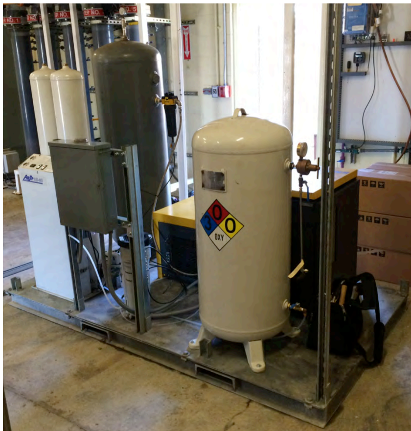
Figure 2.5 - Oxygen generation skid, during installation
