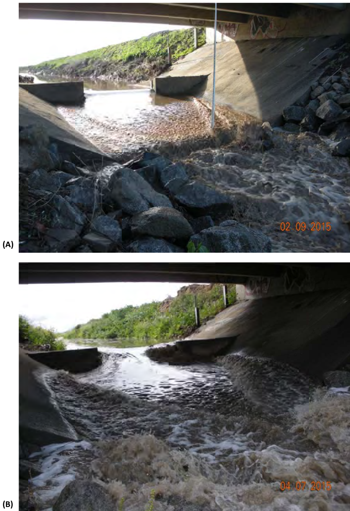
Figure 2: Field images of flow through the San Jon Road weir at flow rates of (A) 30 cfs and (B) 65 cfs.
